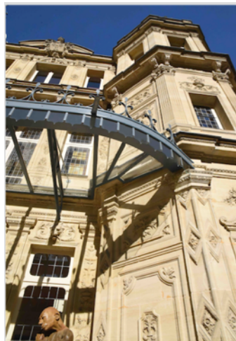
GMDP Architecture – 14 rue Cassette – 75006 PARIS Photo : O Y Lagadec
